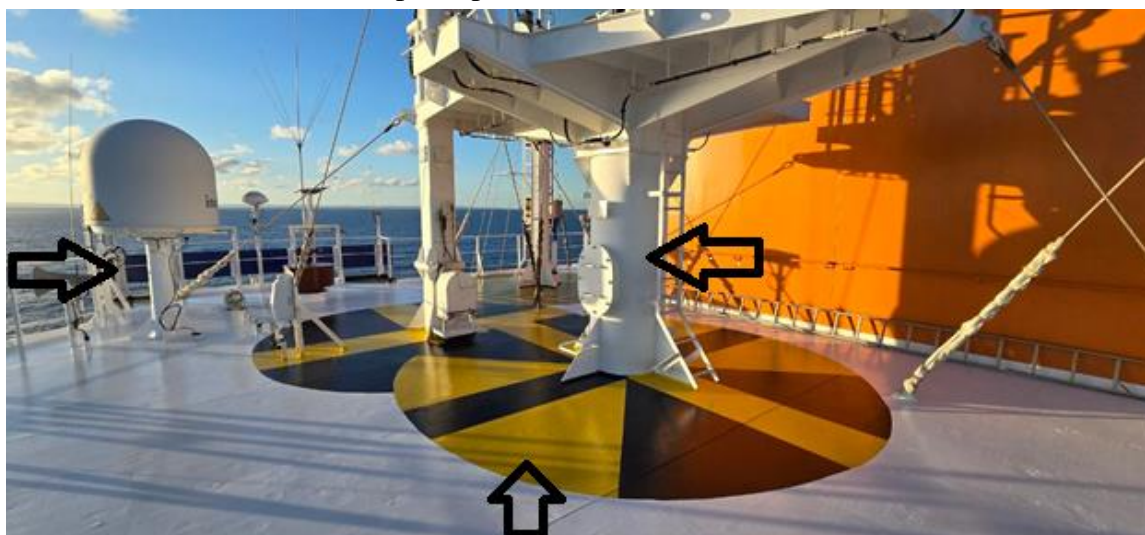
Figure 1 – Navigation equipment of the container ship SPYROS V with applied coatings (arrows show: coating of elements of foundation pedestals for fastening elements of navigation equipment; surfaces for visual identification of dangerous objects that are a source of electromagnetic radiation)
